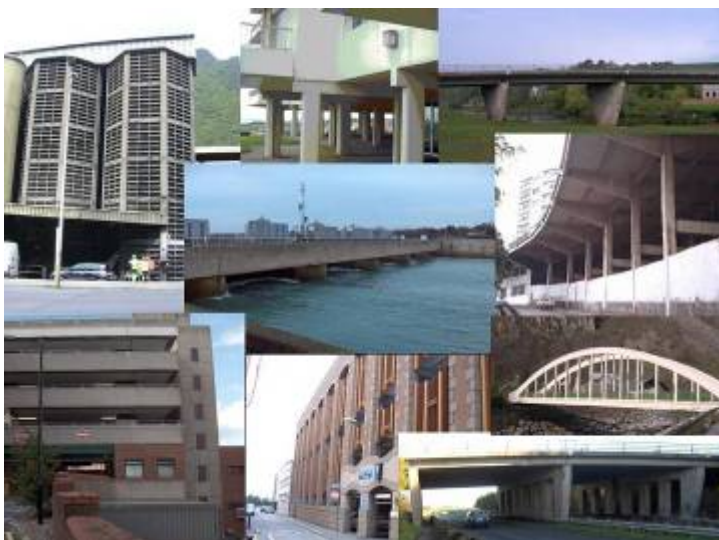
Figure 10 A selection of the structures that have been treated with the hybrid electrochemical treatment.
